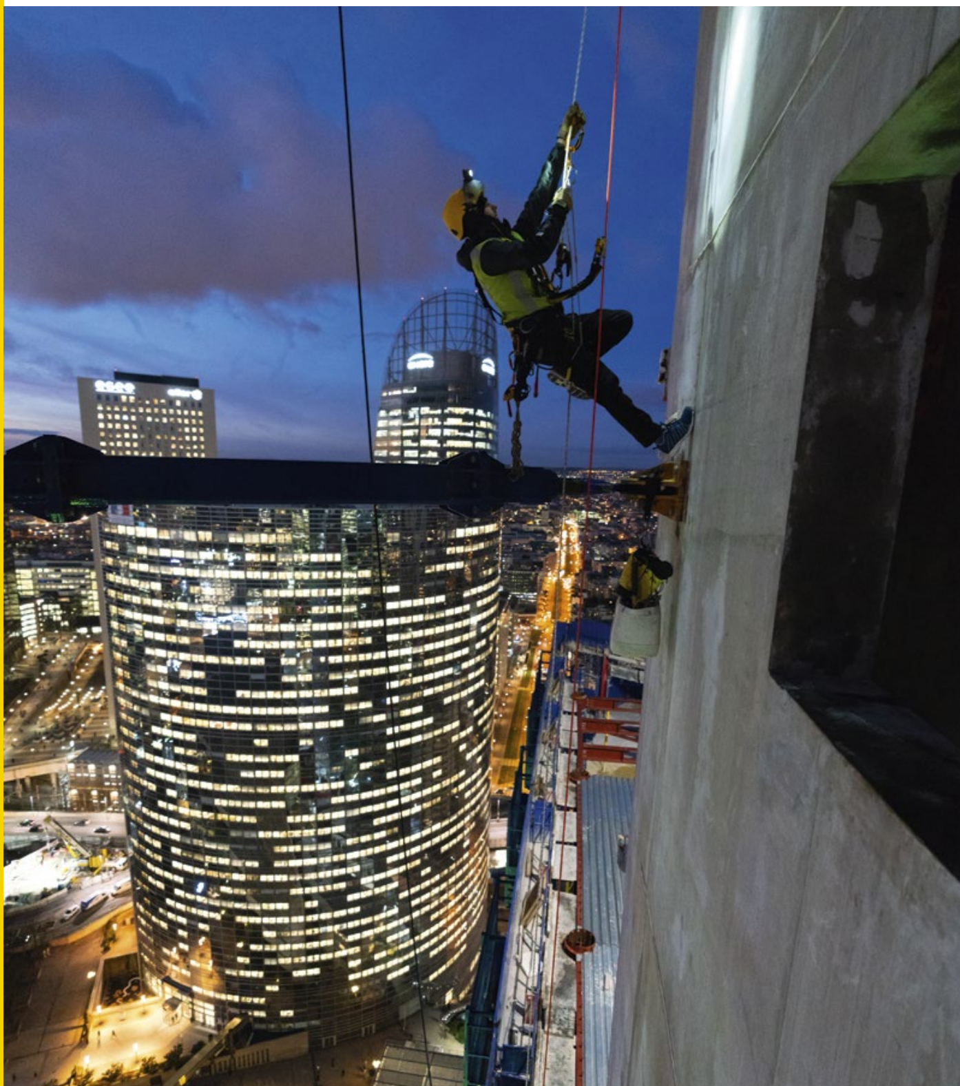
Repositioning the braces of a tower crane, France © 2019 - Petzl Distribution - Vuedici.org - Integral - Bateg - Tour Trinity - Cro&Co Architecture
