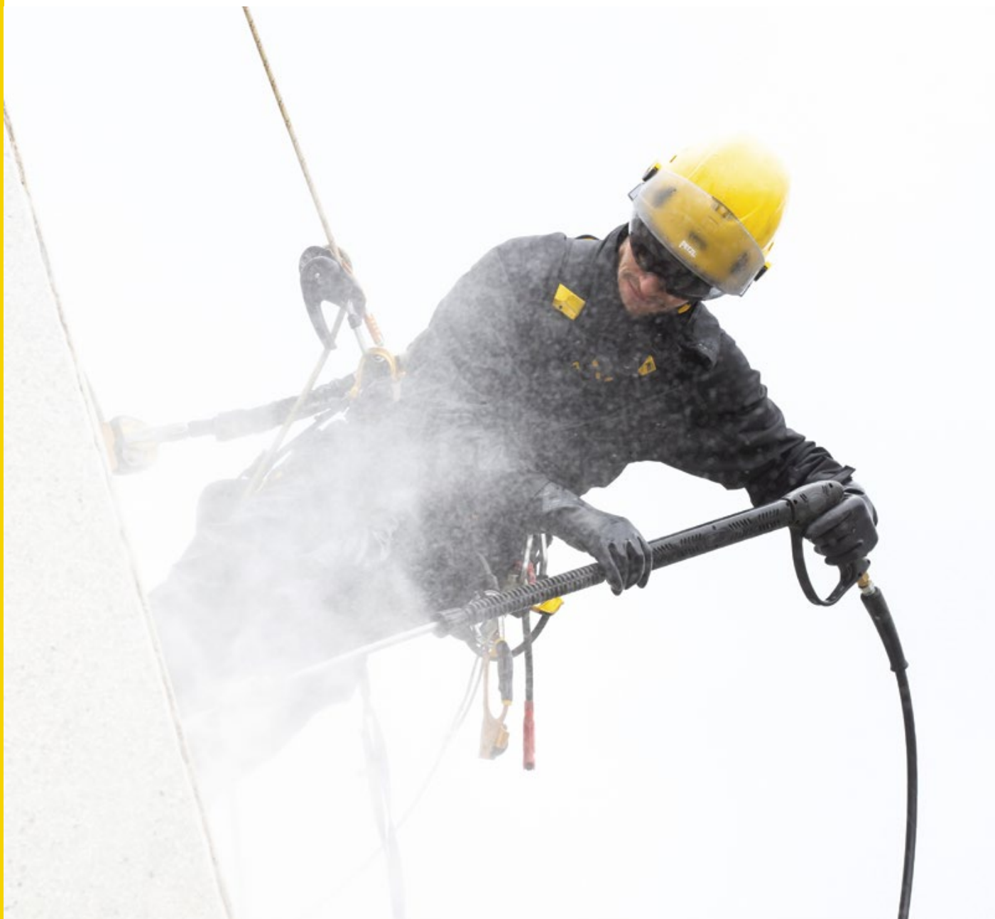
High pressure cleaning of the Petzl solution building © 2019 - Petzl Distribution - Lafouche - Jamias
